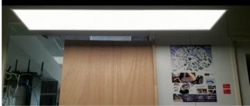
When in Close position, the openable membrane lighting box shows no difference to other normal lighting box.
